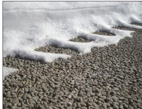
Pervious concrete surface in a cold region
